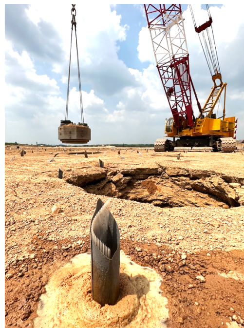
Figure 12 PVD draining through the surface during DC operations
