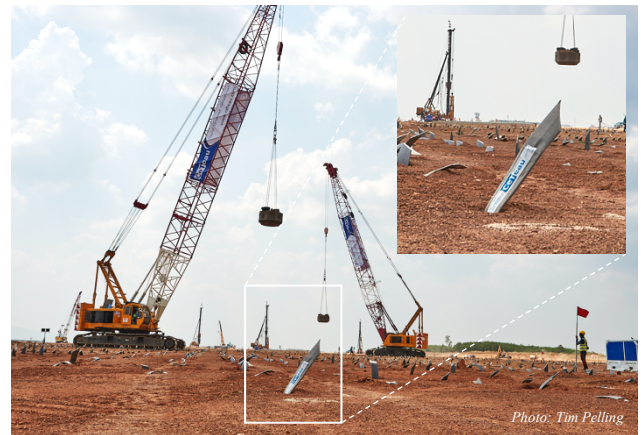
Figure 18 Detail of PVD in advance of Dynamic Compaction
