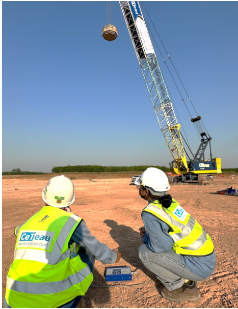
Figure 19 Vibration monitoring during DC works
