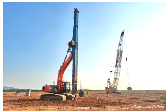
Figure 23 PVD Rig (foreground) and DC Rig (background) at the EV Project
