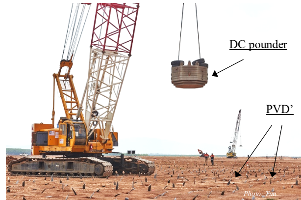
Figure 11 Dynamic Compaction works after PVD’s are installed
