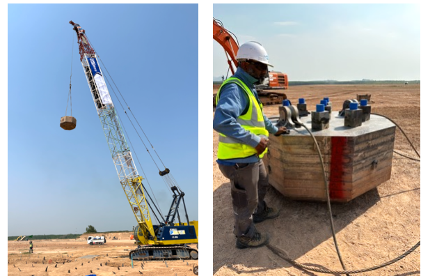
Figure 8 Crane and tampers for Dynamic Compaction
