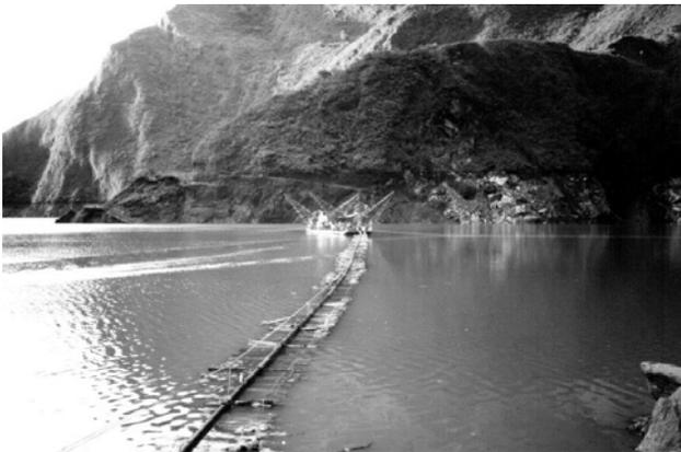
Figure 6. Raft of logs and bamboo supporting steel pipe transporting concrete.
