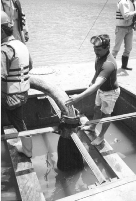
Figure 5. Filling of geotube in cradle.
