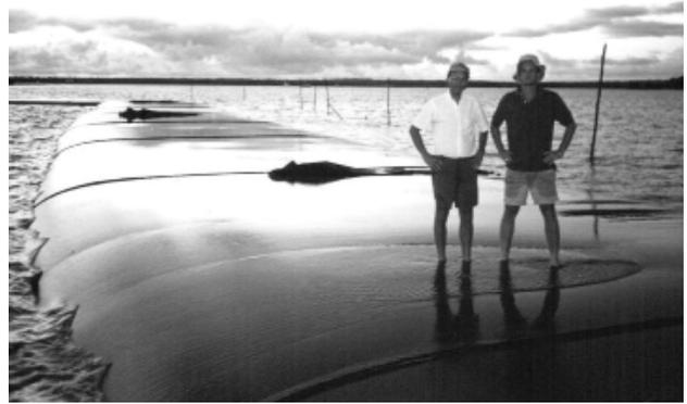
Figure 1. View of geotube being filled.
