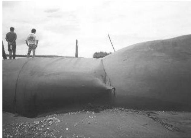
Figure 2. Example of watertight joint with two joining geotubes.
