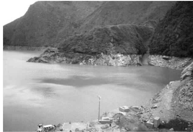
Figure 4. Rock and surficial sediment slides were potential danger to turbines.
