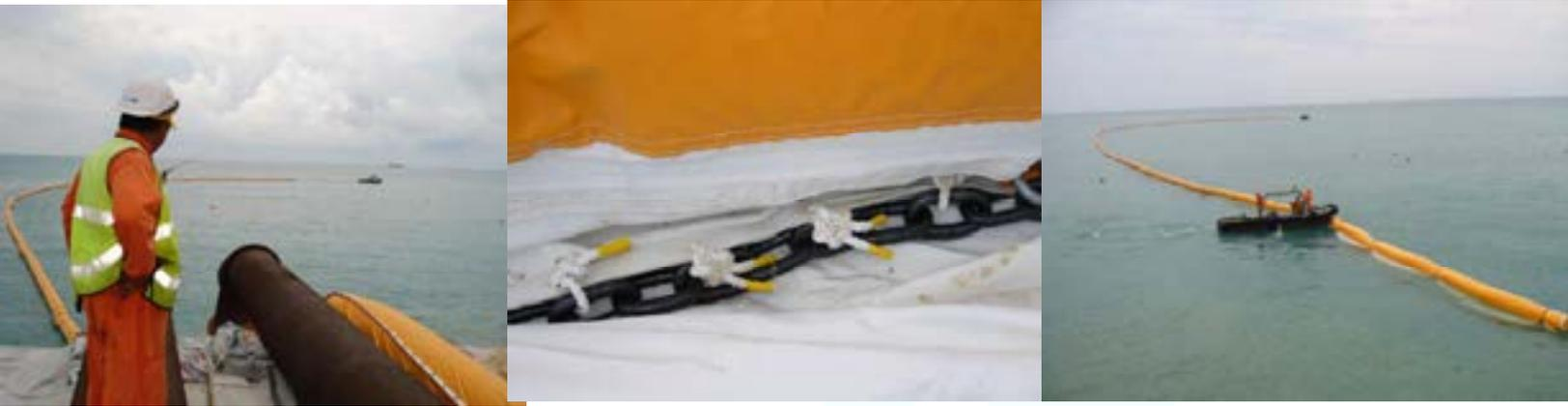
A Silt Protector is a flexible membrane product consisting of woven geotextile that has been designed to physically prevent diffusion of pollution generated in dredging or reclamation works on the seas or rivers.
